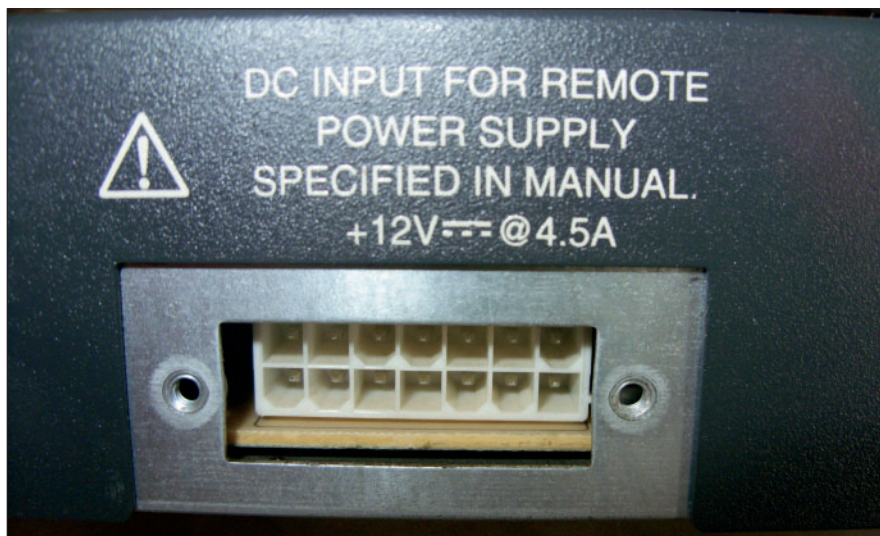
Figure 3-2: A typical 12V power connector for a switch.
